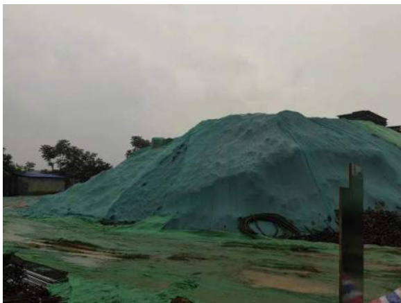
堆土区临时苫盖
